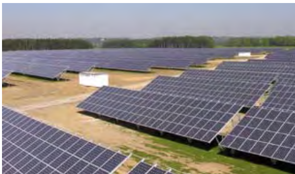
Fig. 1: How many MWh of electricity will this plant generate in a typical year? In order to answer this question, the properties of the installed module type as documented in its data sheet must be modelled as exactly as possible. Each percentage point error in the prediction corresponds to a financial value of about € 35,000 per year for a system with 10 MW installed power (as illustrated here in the photo).
