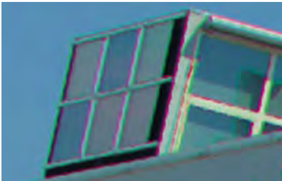
Fig. 2: The same insulating glazing units as in Fig. 1 are viewed here under an incidence angle of 75 °. The colour differences between the different product families are now clearly visible. Such colour differences can be evaluated quantitatively with a colorimetric camera and a measurement and analysis method which was developed at Fraunhofer ISE.
