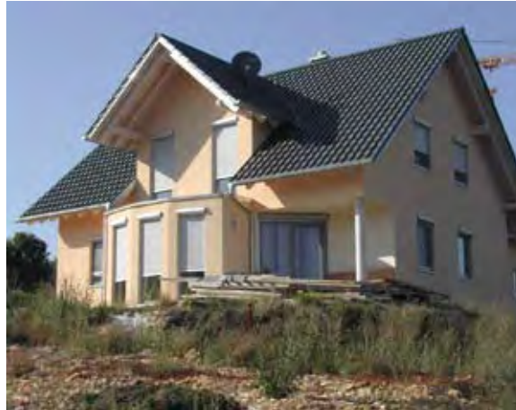
Fig. 1: A demonstration building clad with the 90 mm thick, composite VIP insulating system (free-standing house near Giengen/Brenz). The U value for the wall: U_W = 0.13 \text{ Wm}^{-2}\text{K}^{-1} .
