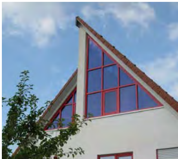
Fig. 1: Switchable gasochromic façade, installed in a building belonging to the company, Werner Herr GmbH, in Ebringen (September 2008). Aspect of the complete façade in the switched state, viewed from the south-west.
