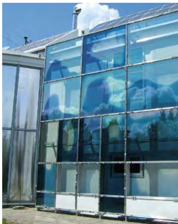
Fig. 2: Switchable gasochromic test façade at the Solarhaus Freiburg (January 2008).
